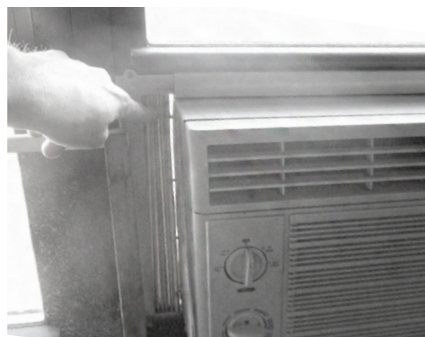
Window AC with air leak at accordion panel
