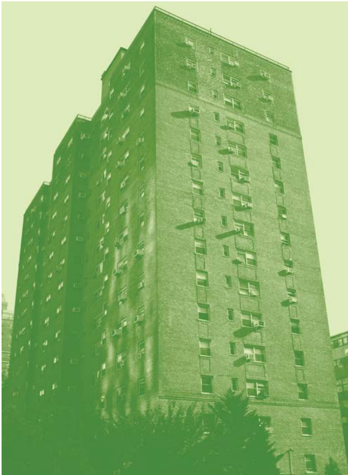
The subject building faces many challenges common to a wide variety of New York City buildings, including masonry exterior walls with no insulation, aging, windows, and merely adequate ventilation.
