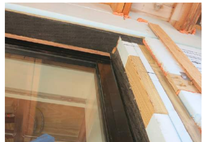
WINDOW INSTALLATION WITH SIGA TAPE & M2 CONTRACTING.
