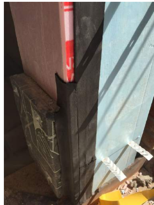
PROVIDING INSULATION WHERE STEEL WAS REQUIRED FOR LARGE MASONRY OPENINGS.
