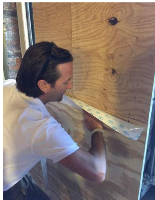
WINDOW INSTALLATION WITH SIGA TAPE & M2 CONTRACTING.
