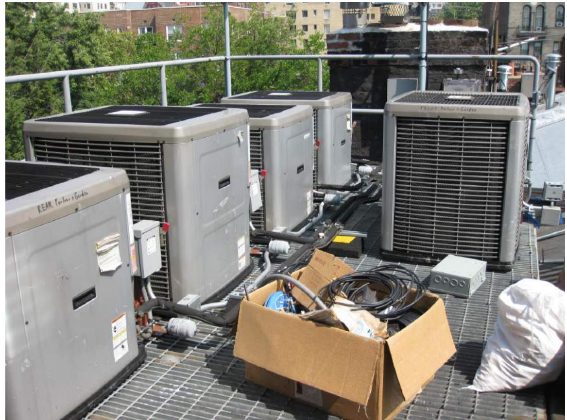
SEVERAL ROOFTOP CONDENSING UNITS
