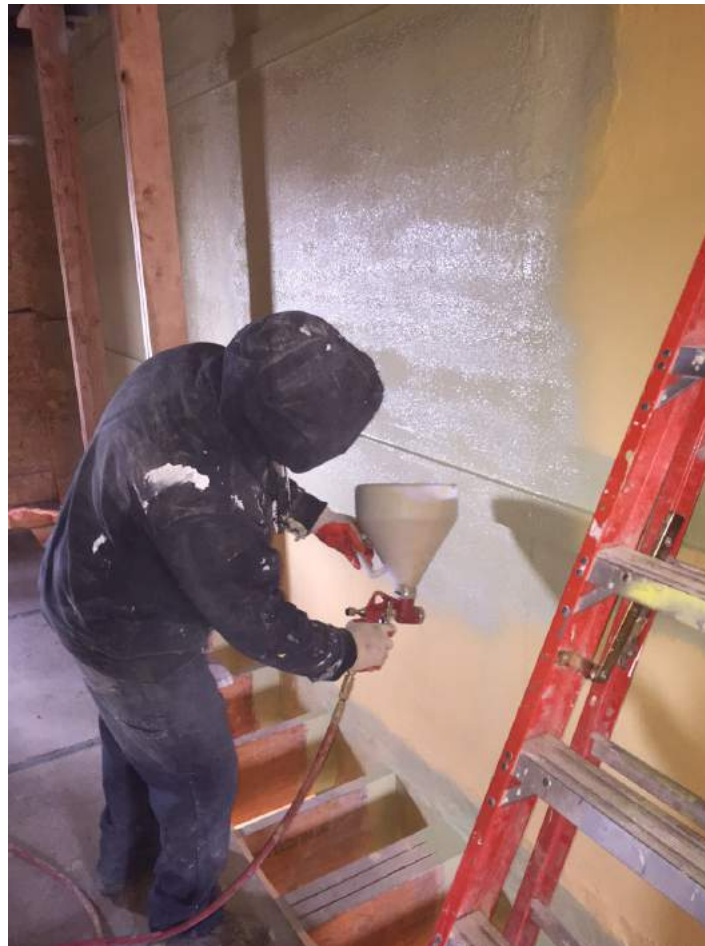
SPRAY STO AND LIME-BASED MORTAR. A PAIR OF SPRAYERS CAN COVER A FLOOR A DAY.
