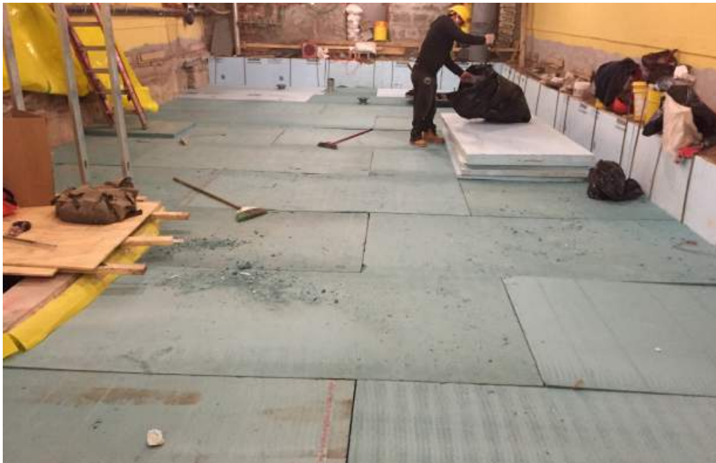
UNDER-SLAB INSULATION
