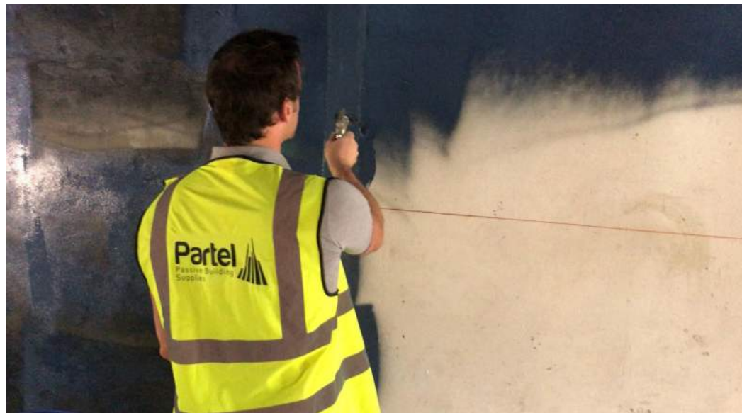
SPRAY APPLICATION BY PARTEL & BRENNAN BRENNAN
