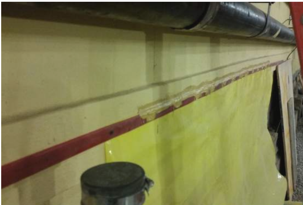
TERMINATION BAR AND STEGO MASTIC DETAIL AT PARTY WALL
