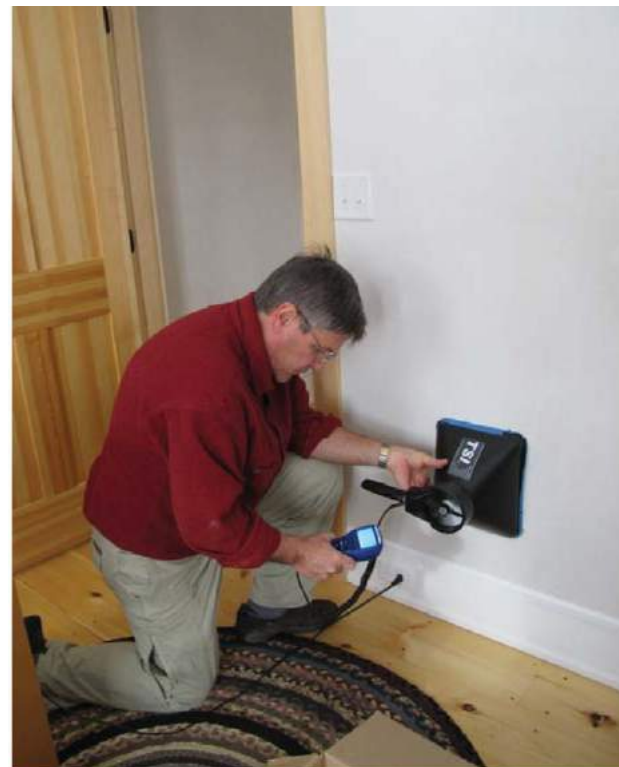
ROUTINE SYSTEM BALANCING ALEX WILSON, BUILDINGGREEN, INC.
