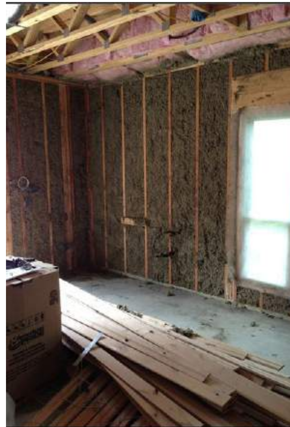
SPRAY-APPLIED ROCKWOOL, R-4 PER INCH (AMERICAN ROCKWOOL)
