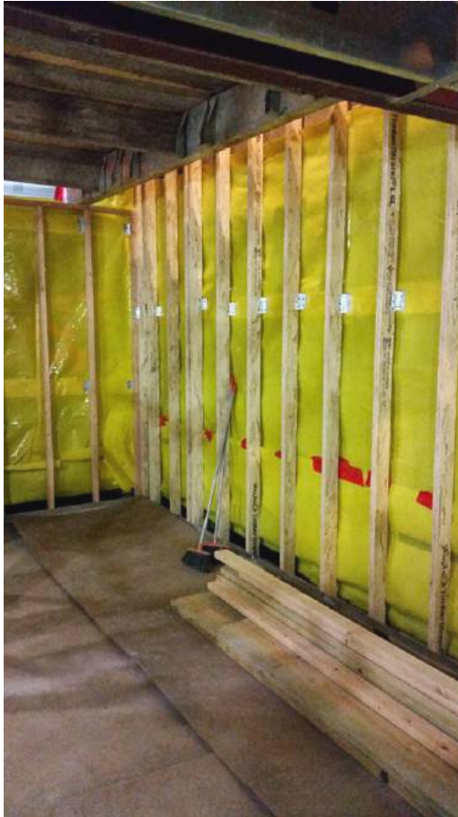
CELLAR PARTY WALL, BELOW GRADE
