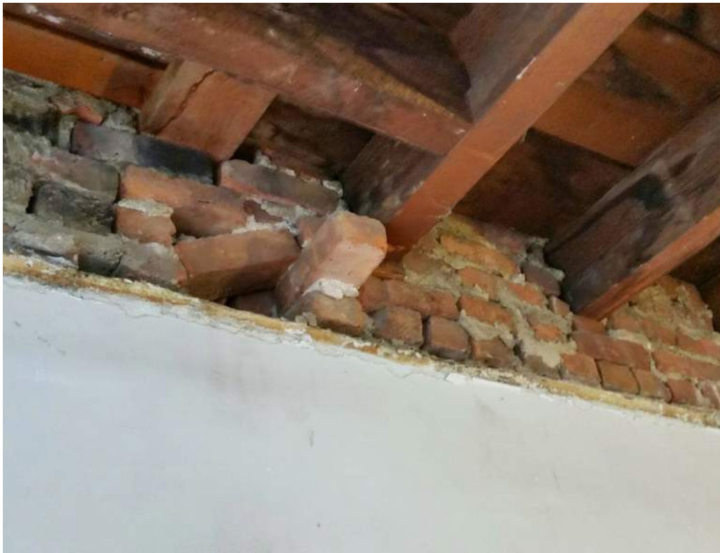
LEFT: TYPICAL TOWNHOUSE FLOOR JOISTS POCKETED INTO THE PARTY WALL.
