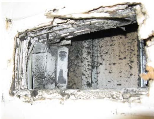
View into a dusty, grimy air duct.
