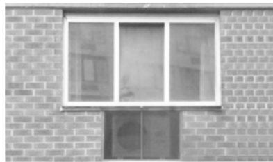
Exterior view of outdoor unit installed under window.
