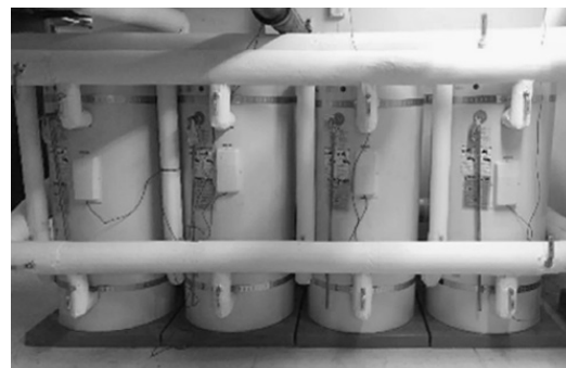
Indoor hot water storage tanks.
