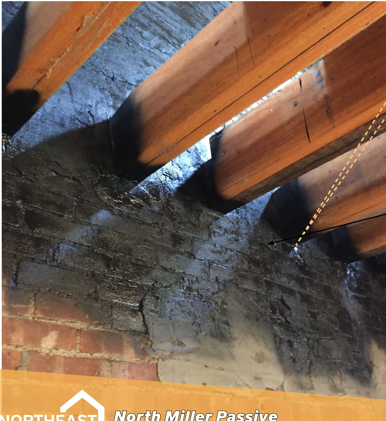
Adhesion on type O plaster - Visconn chips right off
