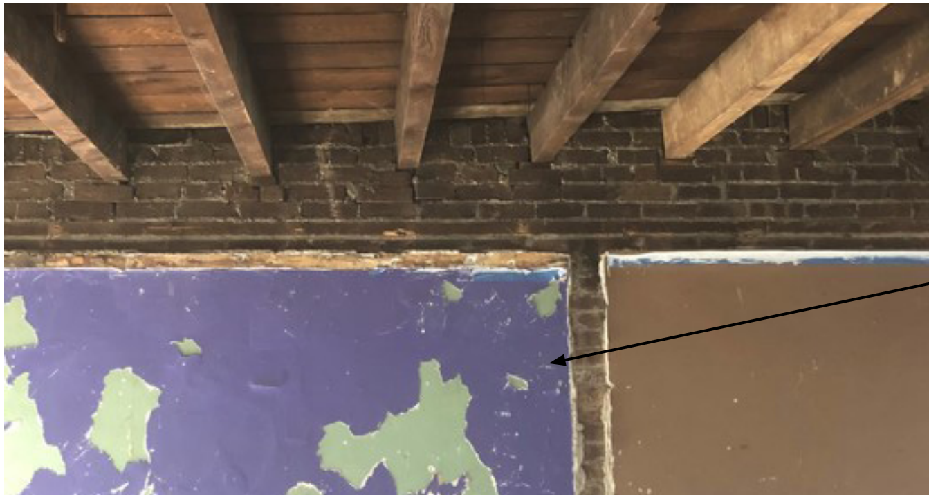
Patches of existing plaster were left
