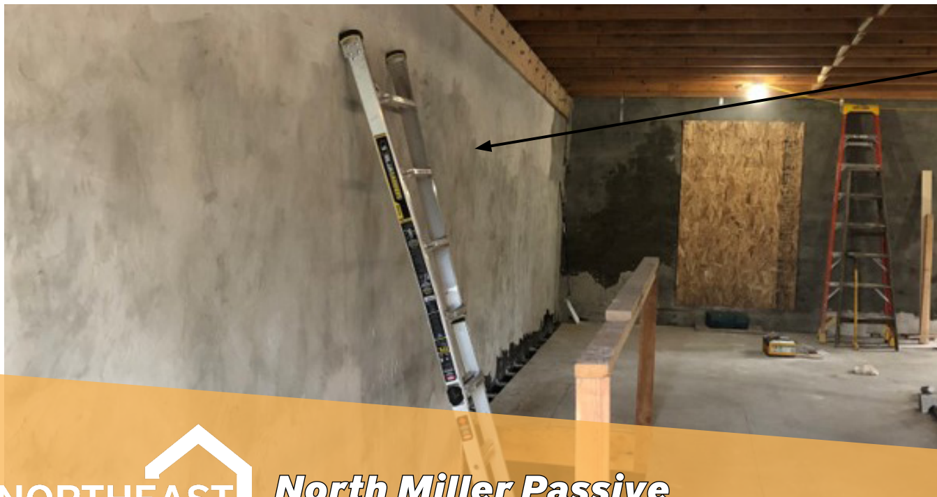
New lime plaster coat
