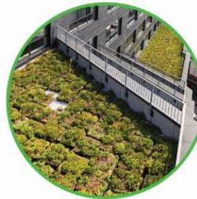
GREEN ROOF TRAY SYSTEM BY CONSERVATION TECHNOLOGY AT SETBACK ROOFS
