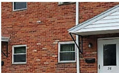
**Existing Window:** Although the frames of high performance windows are typically larger than the existing, the retrofit would allow for the elimination of window AC units, thus increasing the actual daylight area of the windows. Photo Credit: Steven Winter Associates
