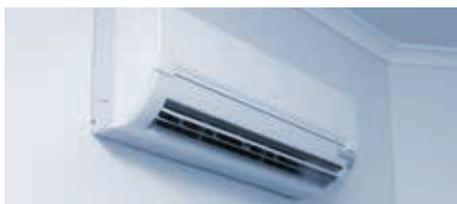
Mini-split heat pump system will utilize interior wall mounted cassettes to deliver both heating and cooling. A unit similar to the one shown here would be installed in each major room, replacing any baseboard heating and window AC units.
