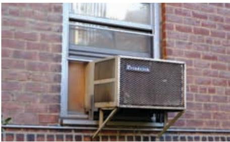
**Existing Window:** Although the frames of the proposed Passive House windows are larger than the existing, because the retrofit would allow for the elimination of window AC units the daylight area of the windows are effectively increased by about 15%. Photo credit: Building Energy Exchange
