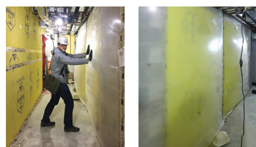
A guarded blower door test in action at Flow Chelsea. Each test measured the exterior air leakage from a single floor in the building.
