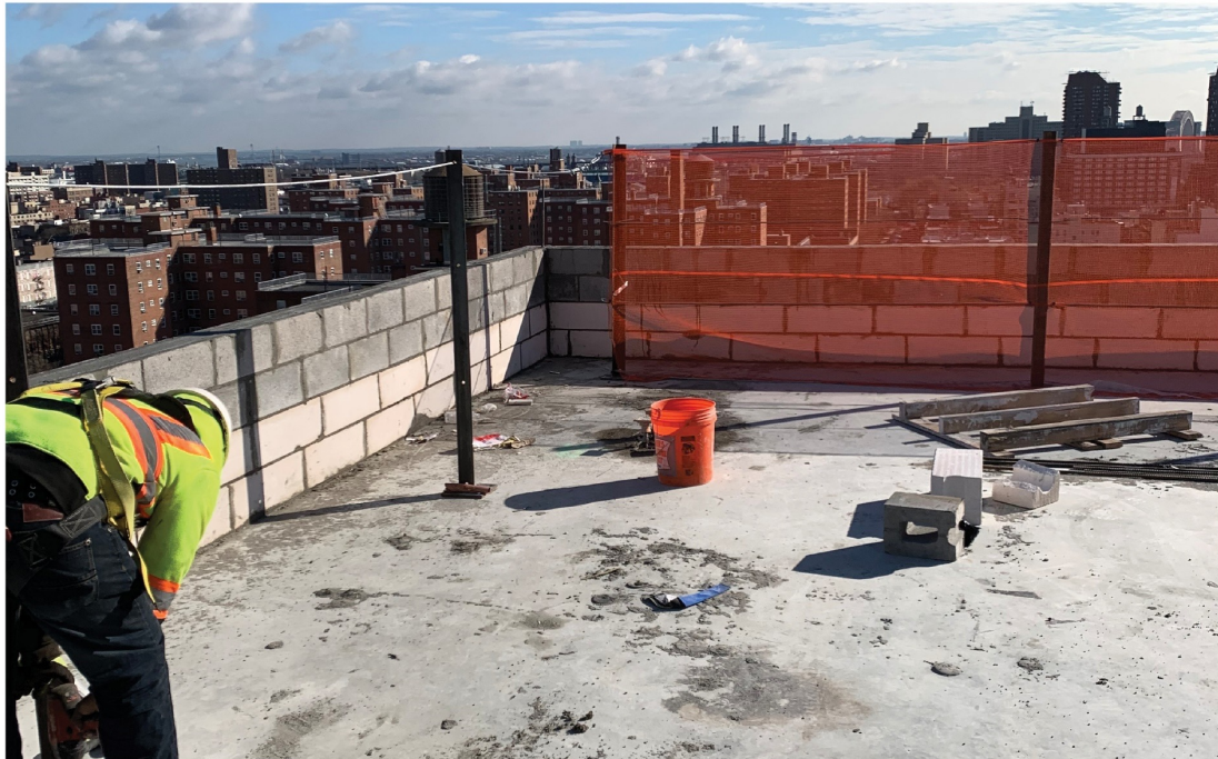
AAC BLOCK @ PARAPETS
