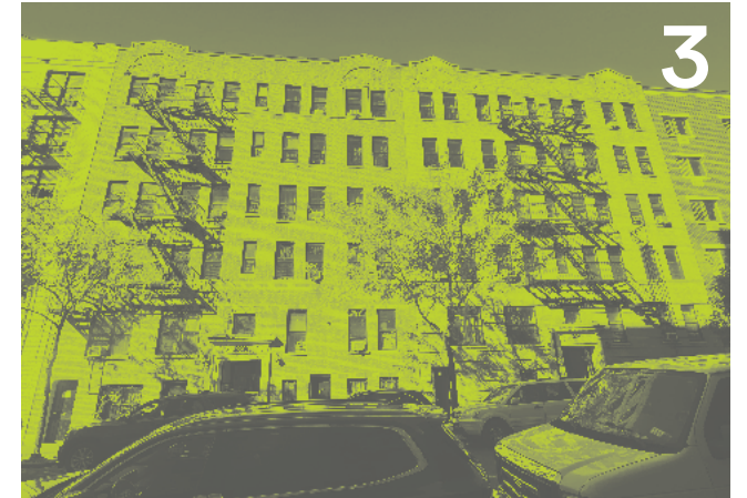
pre-war low-rise rent stabilized rental
