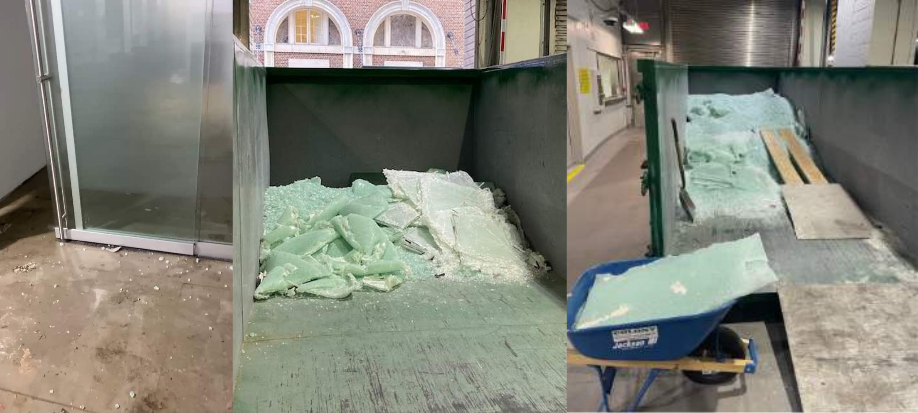
Loading Dock, One Bryant Park BoA Tower
